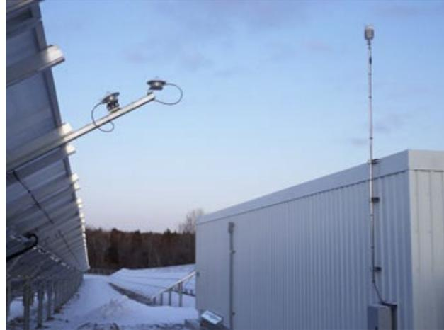
*This weather station installation shows the two radiation sensors, one at plane of array and one at GHI, as well as the Orion weather sensor module on the mast. MicroServer and Acromag amplifier are in the weatherproof enclosure mounted below the mast. Photo courtesy of Industrial Electrical Contactors Ltd.*
